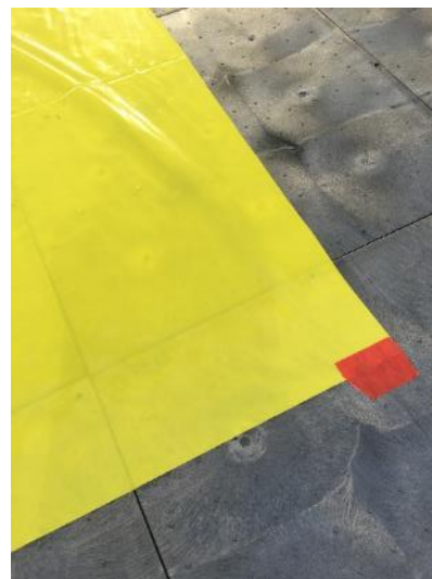
2. Impermeable sheeting prevents contamination of underlying artificial turf
