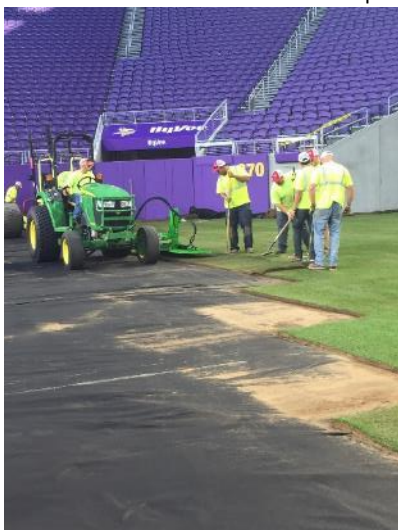
5. Installation of big roll turf
