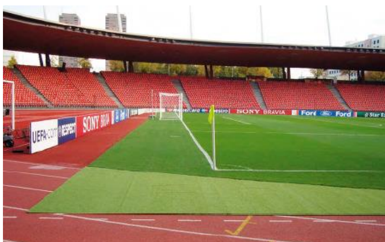
Fig. 2. Extension of turf perimeter around the Field of Play using high quality artificial turf
