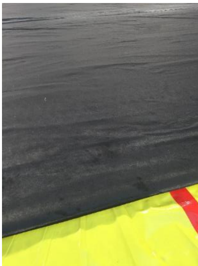
3. Surface is then covered with shockpad
