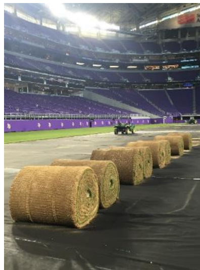
4. Big roll natural turf is delivered
