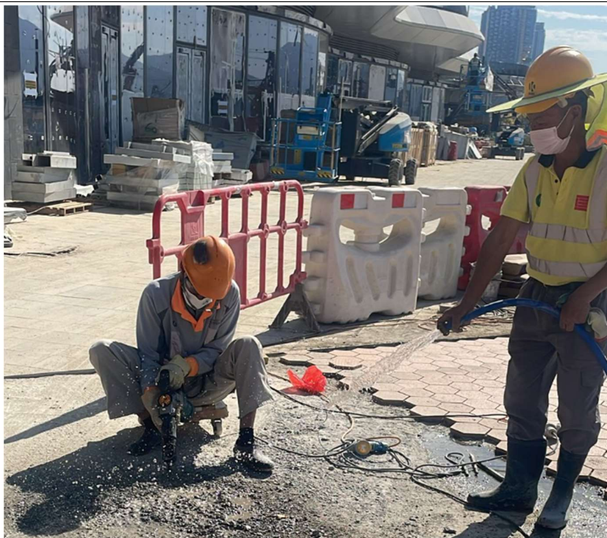
Photo 7: Water spraying had been provided for dust generating works.
