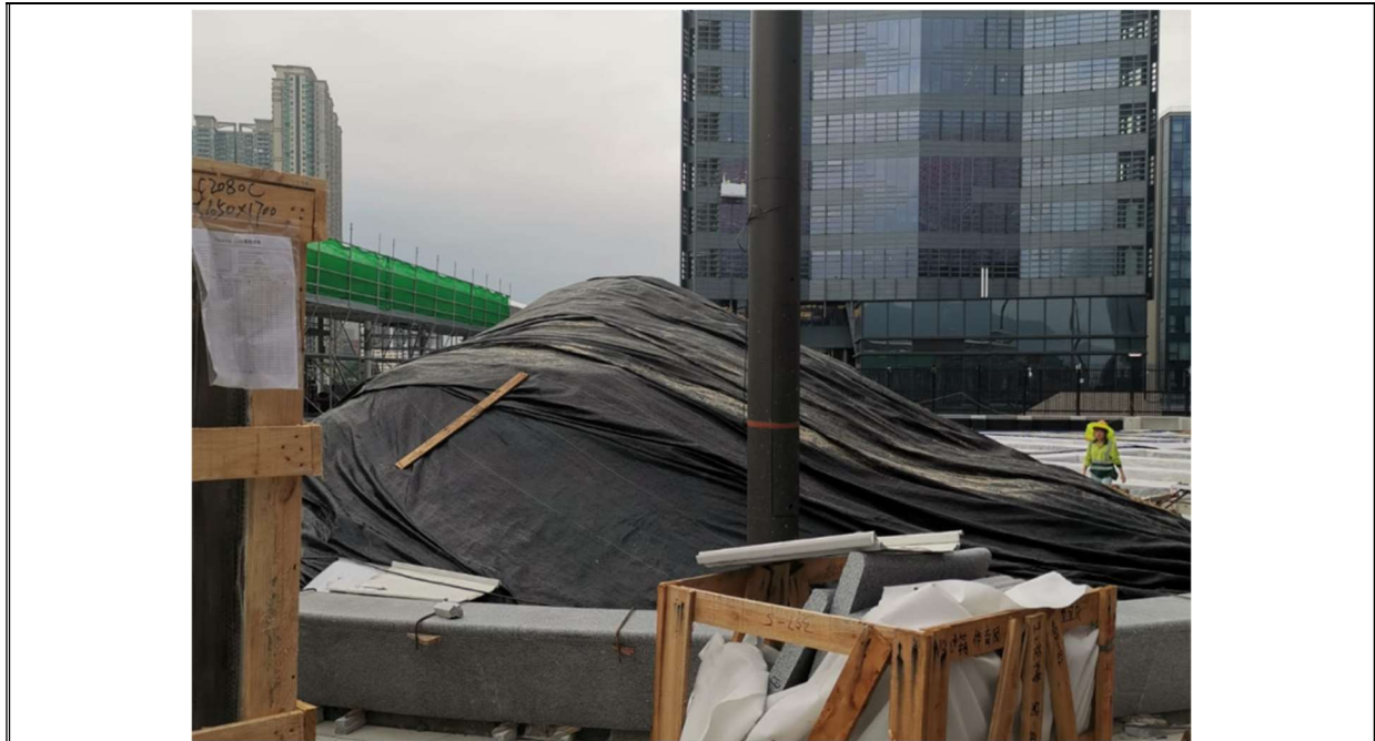
Photo 8: Covering sheet has been provided for stockpile on site.
