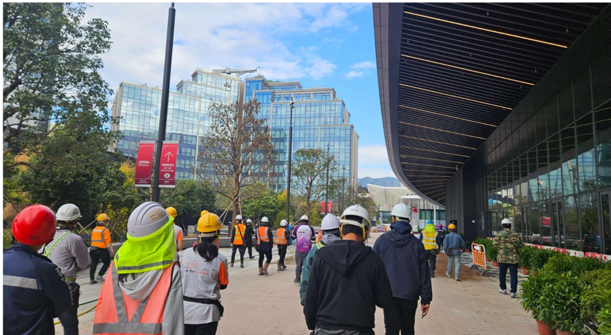
Photo 1: Regular site inspection carried out with contractor on 15 January 2025.
