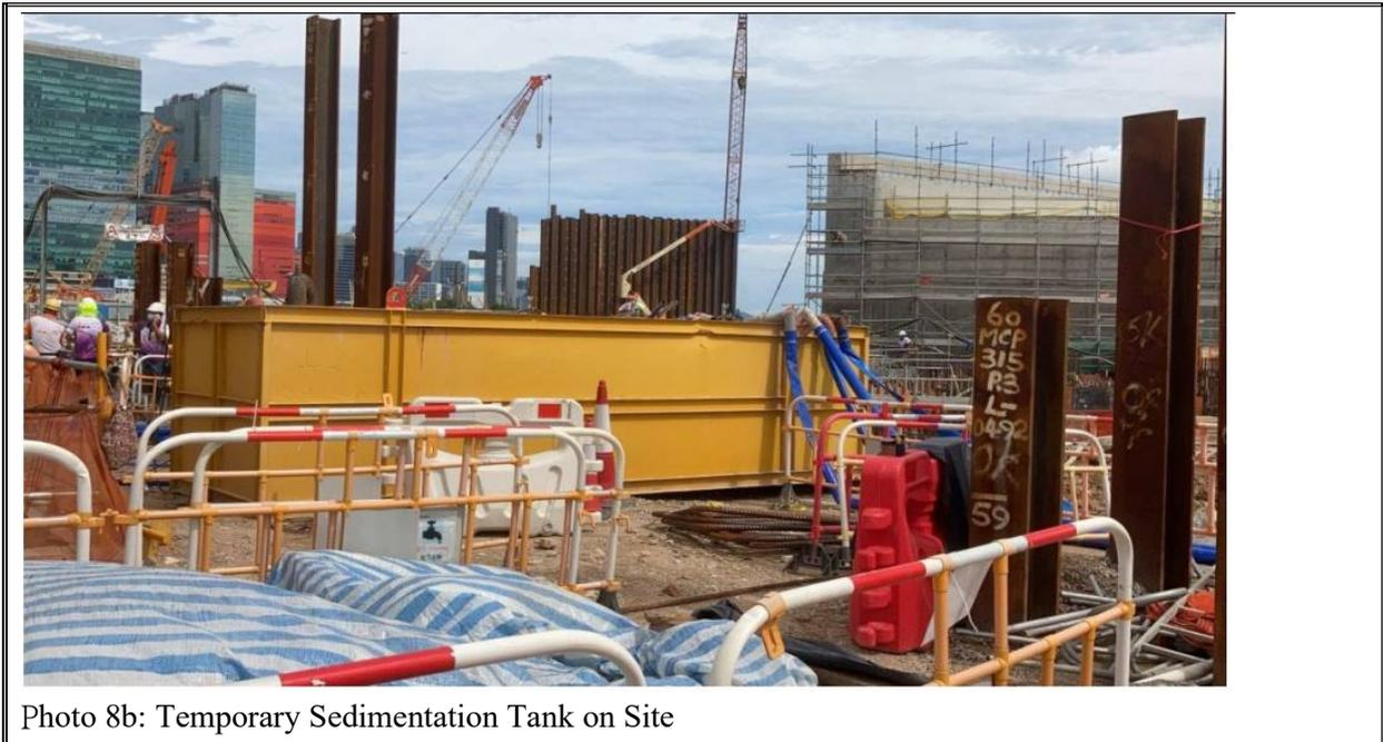
Photo 8b: Temporary Sedimentation Tank on Site
