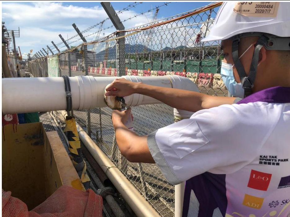
Photo 6a: Regular Sampling at Wastewater Treatment Tank Discharge
