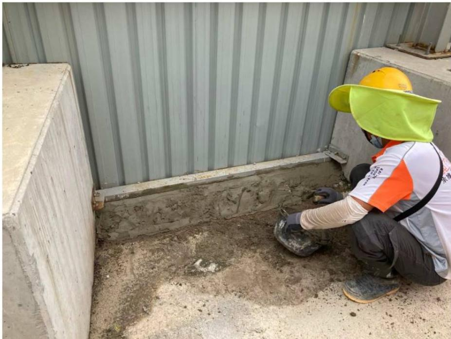
Photo 5: Re-sealing of Footing at Site Hoarding
