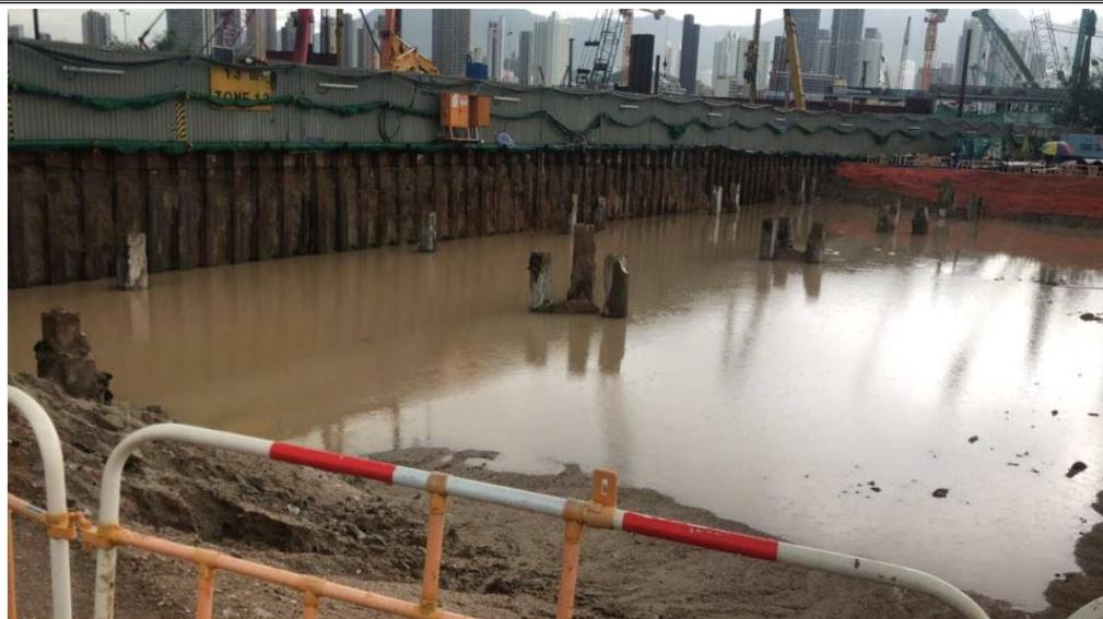
Photo 8a: Temporary Sedimentation Pond on Site
