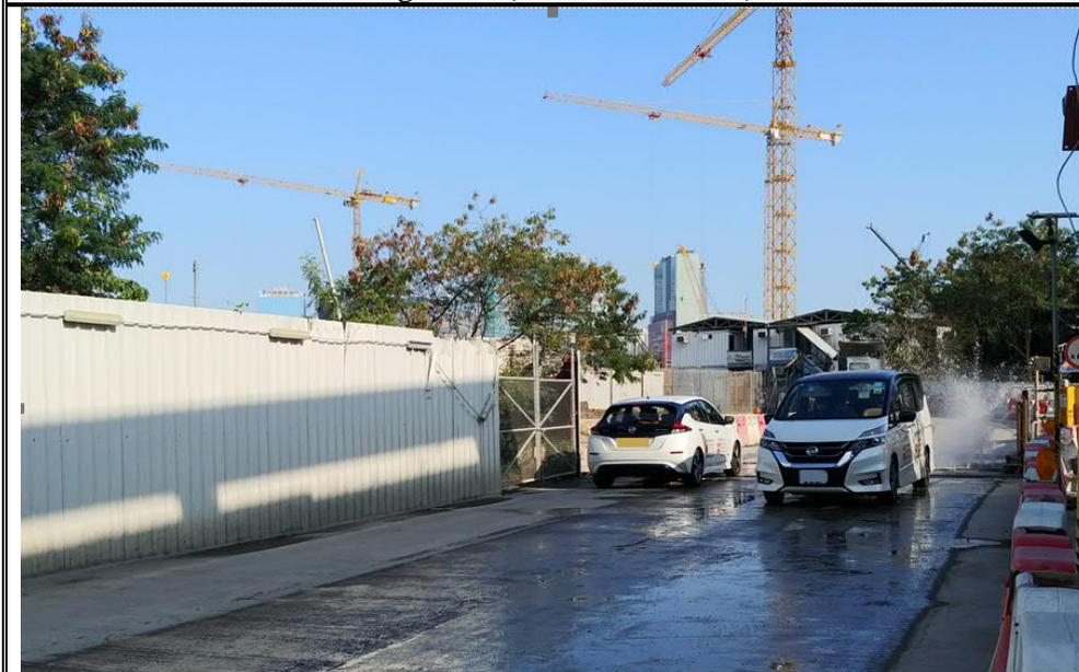
Photo 2: Wheel washing facilities had been implemented for the passage of construction vehicles at gate 3C (1 December 2020)
