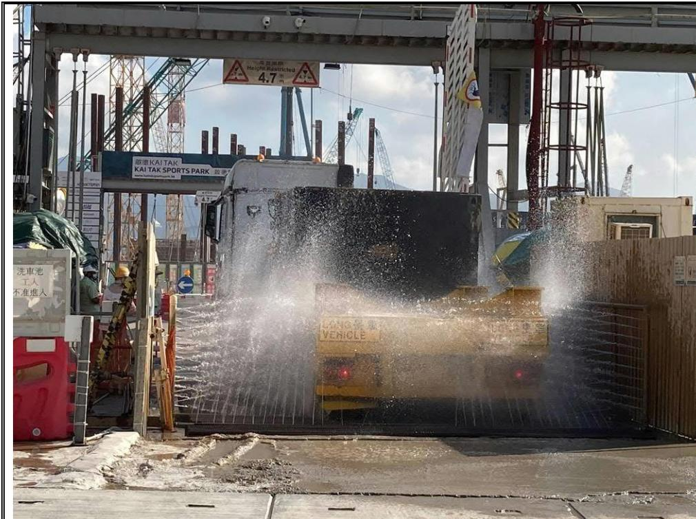
Photo 3b: Wheel washing facilities had been implemented for the passage of construction vehicles at northern gate
