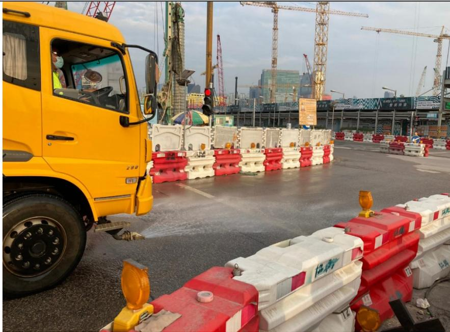
Photo 3: Water spraying truck to wash the road surface at Shing Kai Road (8 December 2020)
