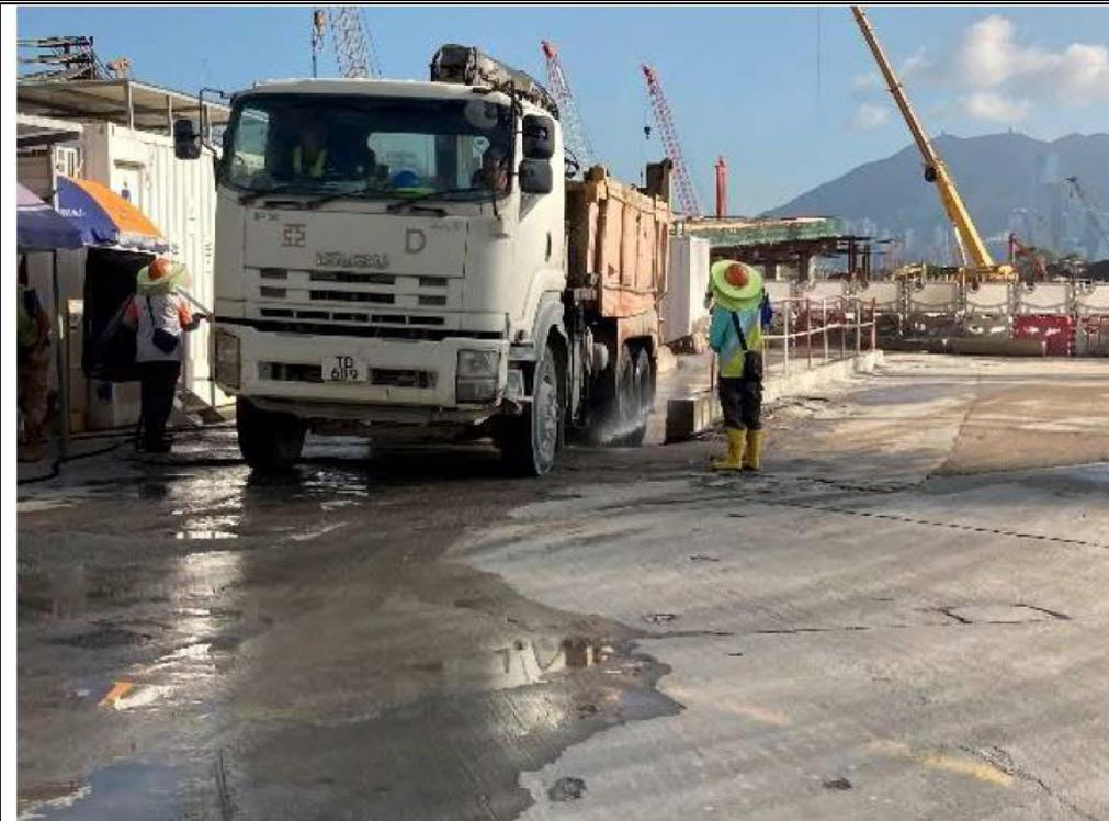
Photo 3a: Wheel washing facilities had been implemented for the passage of construction vehicles at southern gate
