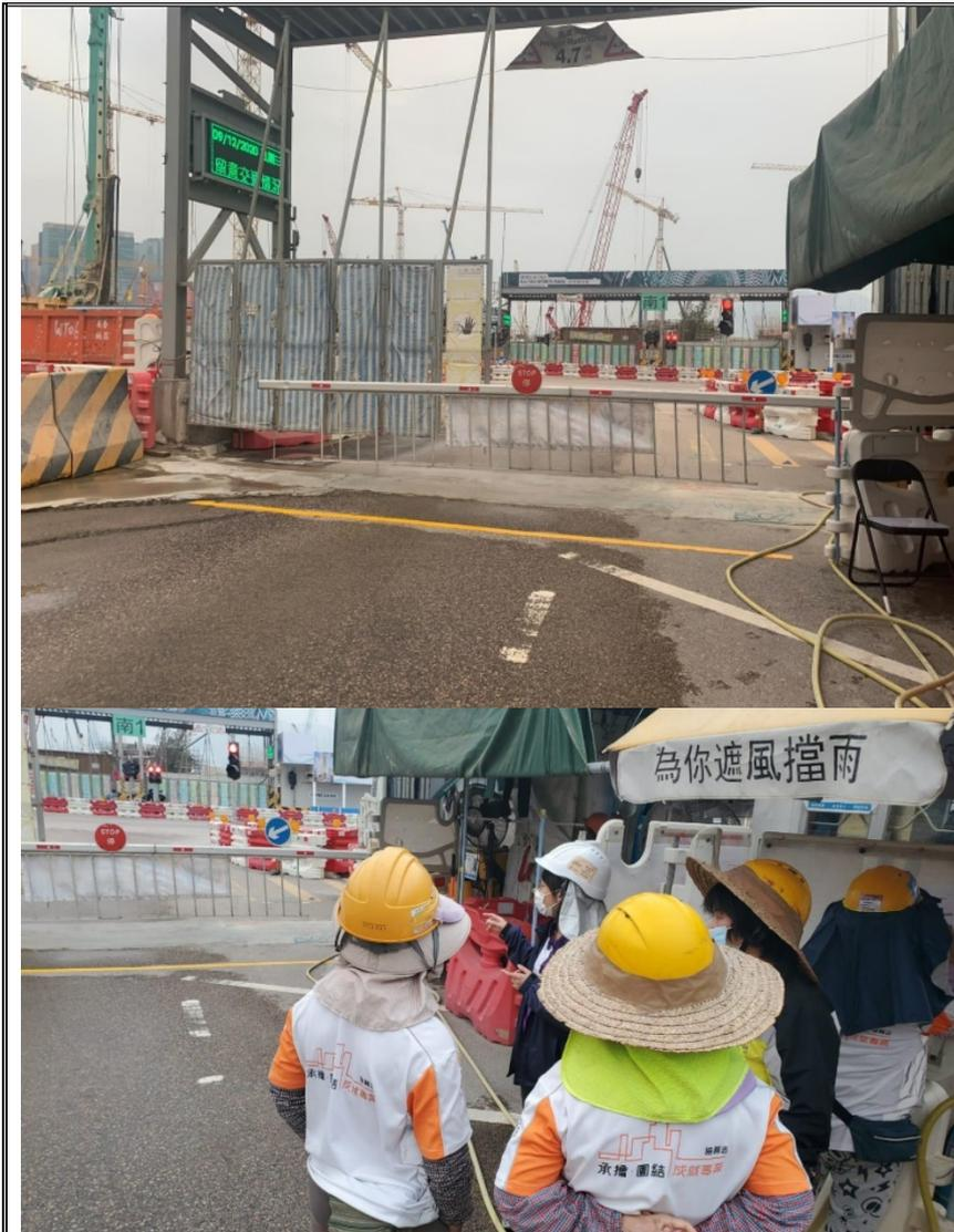
Photo 5a & 5b: Contractor set up yellow line marker at Gate N1 and instructed the workers to provide washing within the yellow line area and to prevent water jetting directing to the Shing Kai Road
