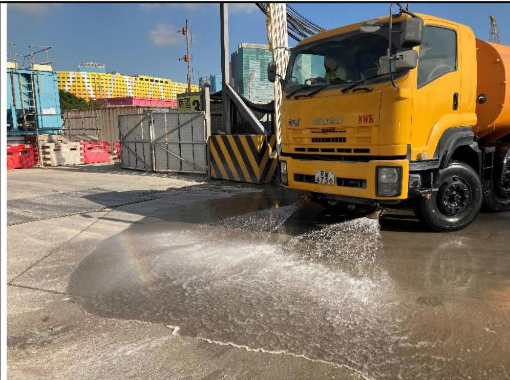
Photo 5: Water spraying truck routinely washes the main haul road and public road to maintain wet surface
