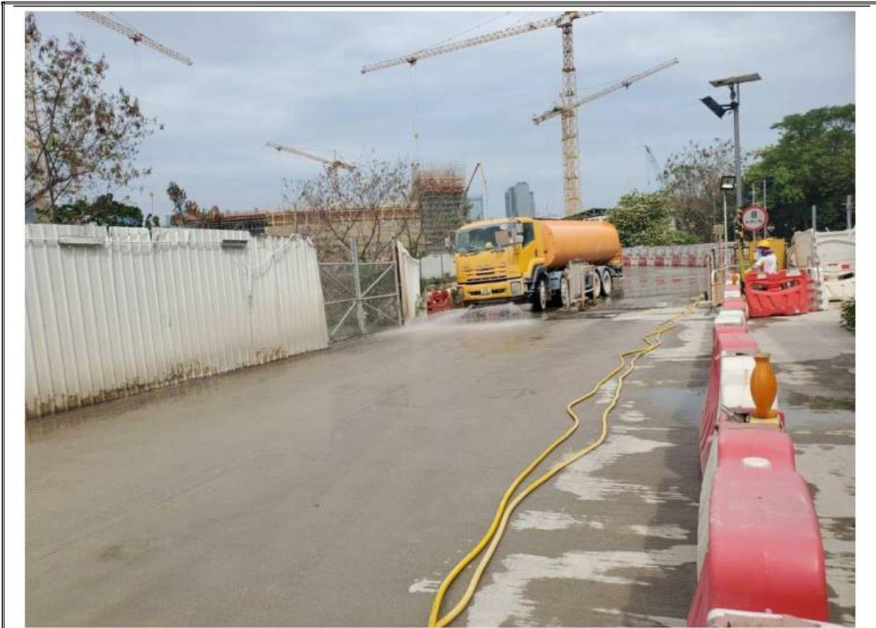
Photo 3: Water truck has been provided regularly at road 3C to remove all dusty material. (16 April 2021)
